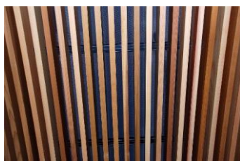
2. Megasorber PN5: acoustic backing for aluminium battens:
