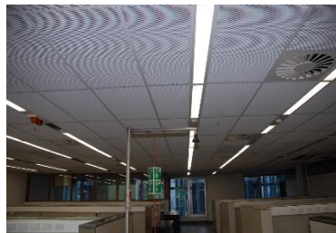
4. Megasorber PN on standard ceiling grids and expanded metal ceiling panels
